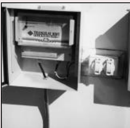
TriangularwaveTechnologies, Inc. Microprocessor installed in a weatherproof electrical box on the outside wall of the building.
